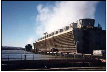
Figure 4–5. Visible Plume
