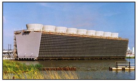
Figure 4-2. Multi-cell Mechanical Draft Cooling Tower
