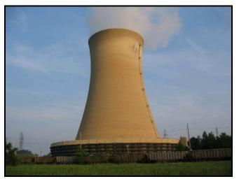
Figure 4-1. Natural Draft Cooling Tower
